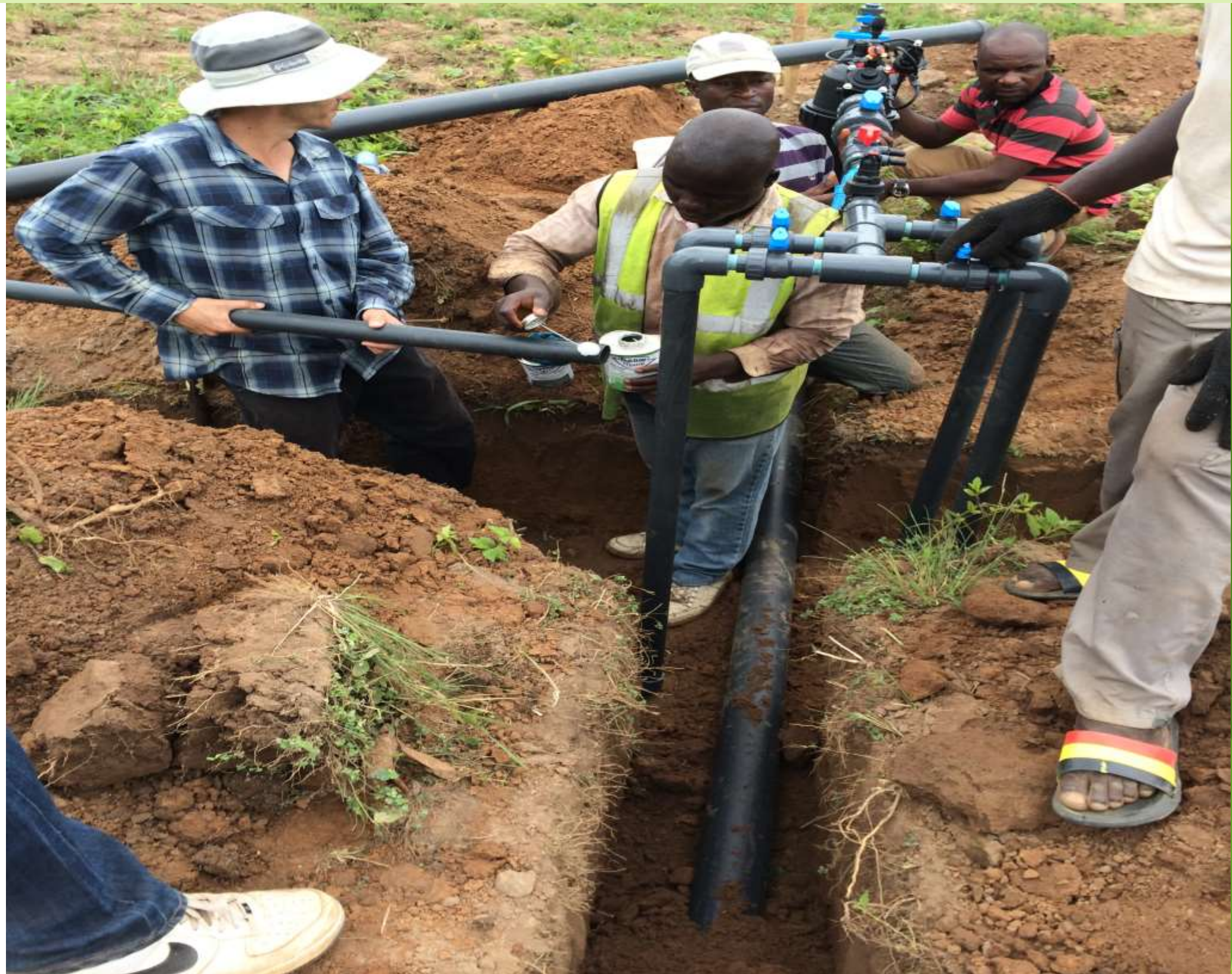
Pipes Laying/Installation
