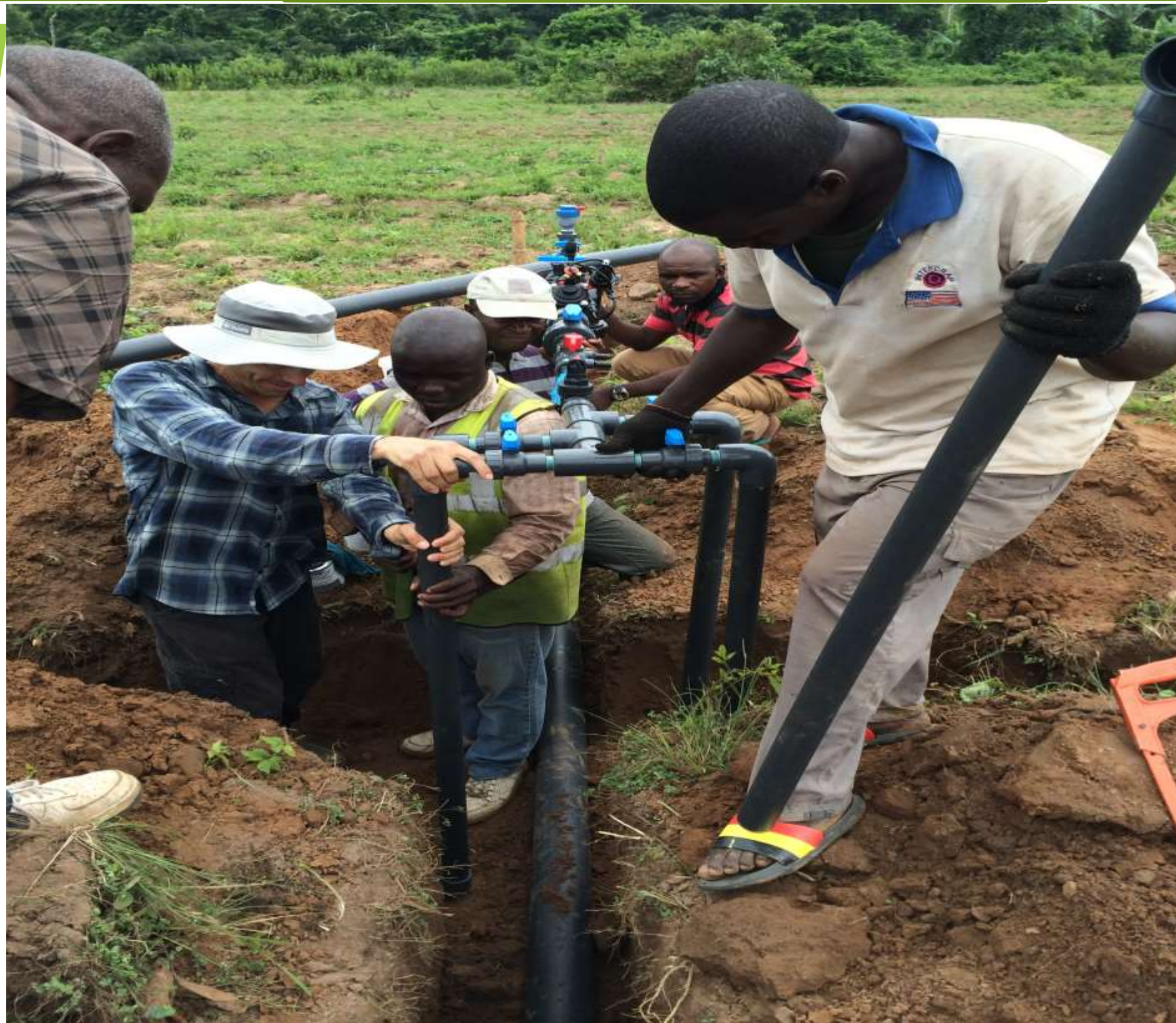
Pipes Laying/Installation
